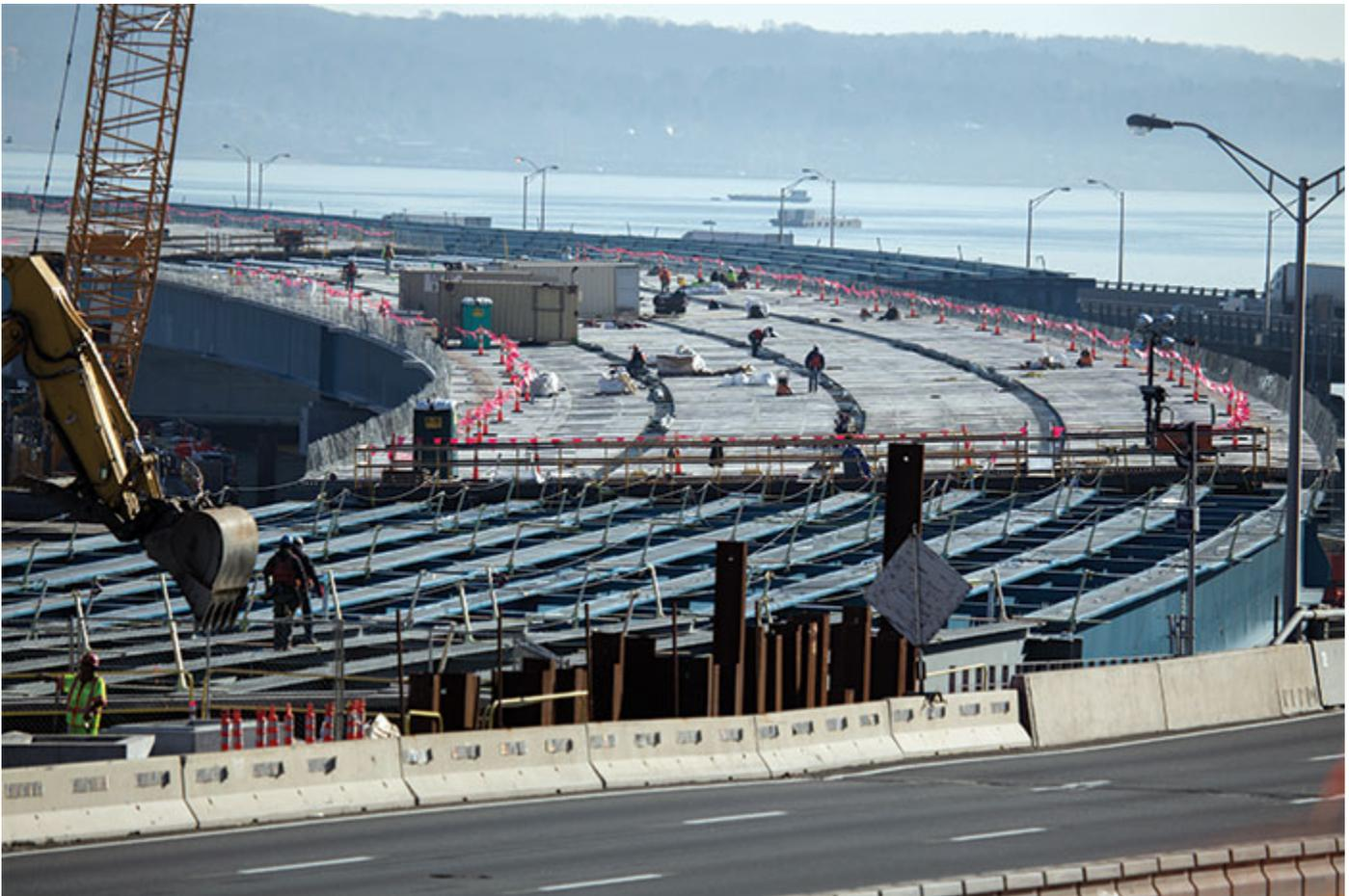
Thirty miles of steel girders for a new highway bridge rising over the Hudson River near New York City are being delivered on a roundabout route using trucks, barges and ports with the space to handle the big cargo.
